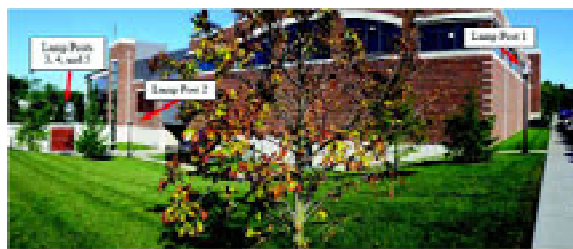
Five lights surrounding the RecPlex are now solar powered.
