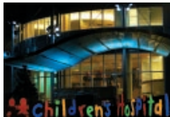
Vanderbilt Children's Hospital, Nashville, TN, Chapel Electric
