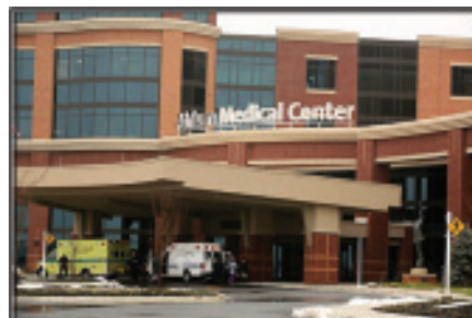
Atrium Medical Center
