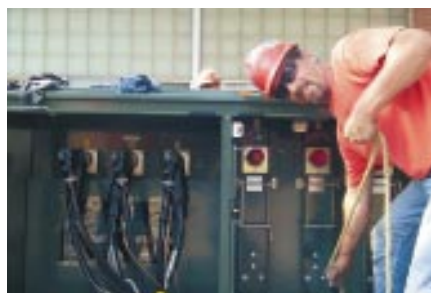
Journeyman Foreman Shawn Stamps, Wagner Smith Electrical
