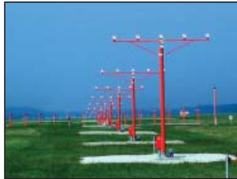
New runway lights installed at WPAFB by ESI.
