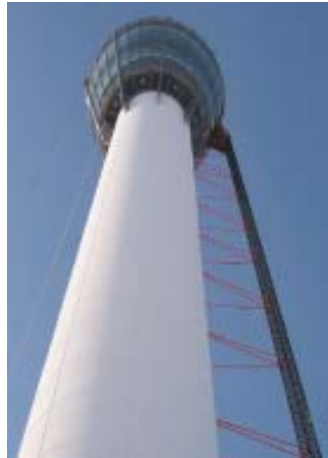
Maxwell Lightning - Air Traffic Control Tower, Indianapolis.
