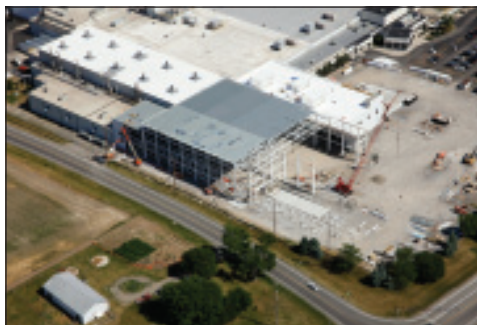
Honda Transmission plant expansion.
